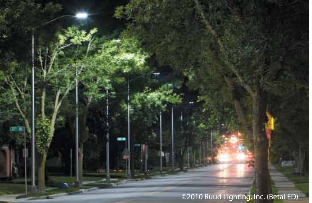
LEDway streetlight with 60 LEDs, Type III medium optics, 525mA, Installed on 39th Avenue, Color Temperature: 6000K
