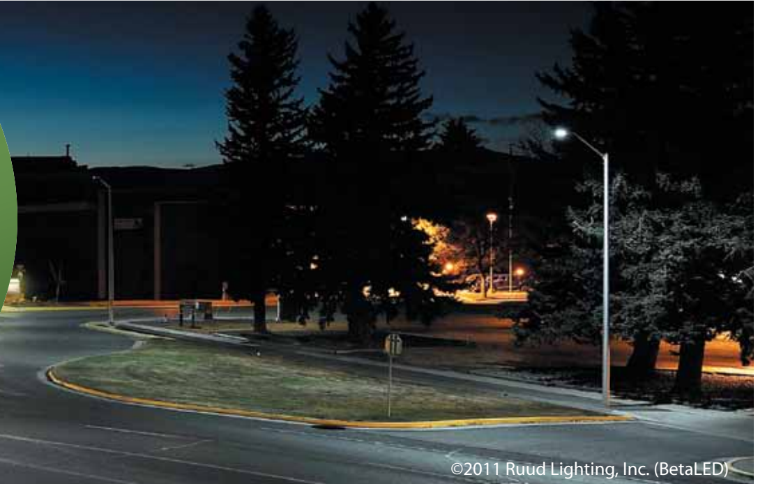
LEDway Streetlights with Type II medium optics, some with backlight control, Color Temperature: 4300K
